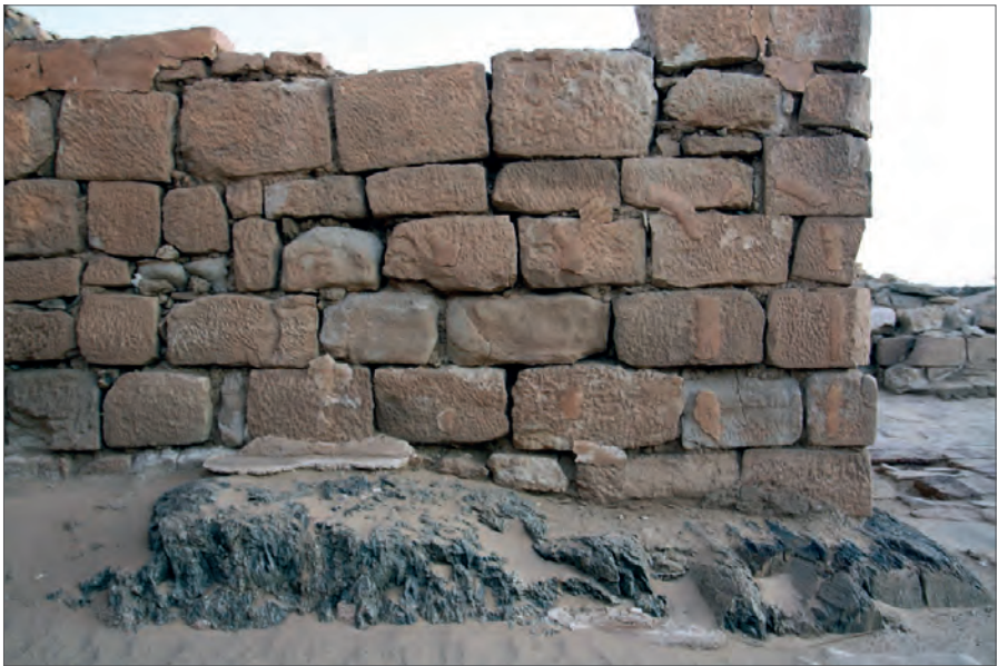
Fig. 15. Plaster in the western bay of the North Church at Ghazali in 2011 (Photo A. Obluski @ PCMA UW)
