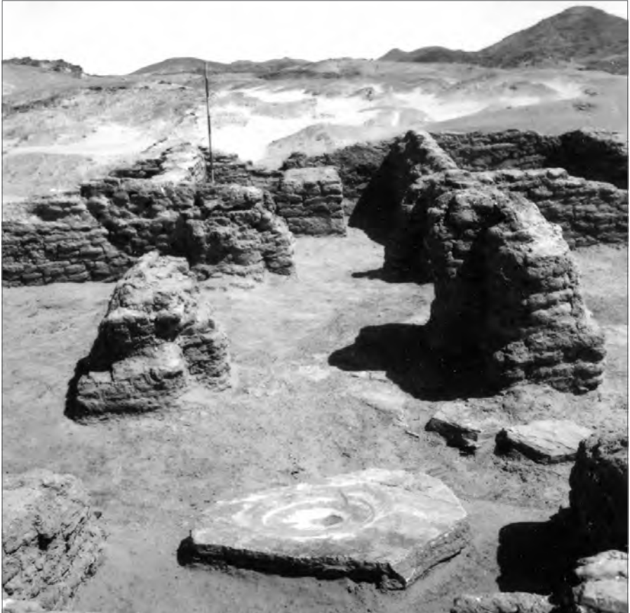
Fig. 12. Church at Duweishat East [16-S-1]. View east towards the altar. Note reused New Kingdom grindstone in the floor in the foreground (Photo ASSN F363/4)
