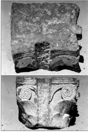
Fig. 7. Slots to mount the wooden screen into the northern column of the triumphal arch, top and side views (Courtesy of the Oriental Institute Archives)
