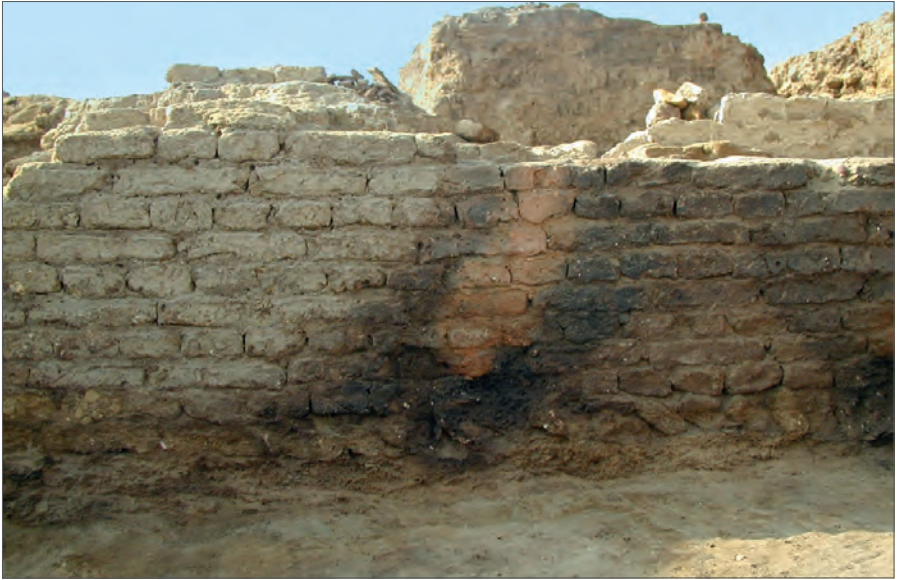
Fig. 3. Burnt patch on the northern face of the south wall of Room D.8, view looking southwest (Photo W. Godlewski © PCMA)
