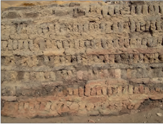
Fig. 23. Traces of burning on the western face of the east wall of Room J.3, view looking east (Photo S. Mašlak © PCMA)
