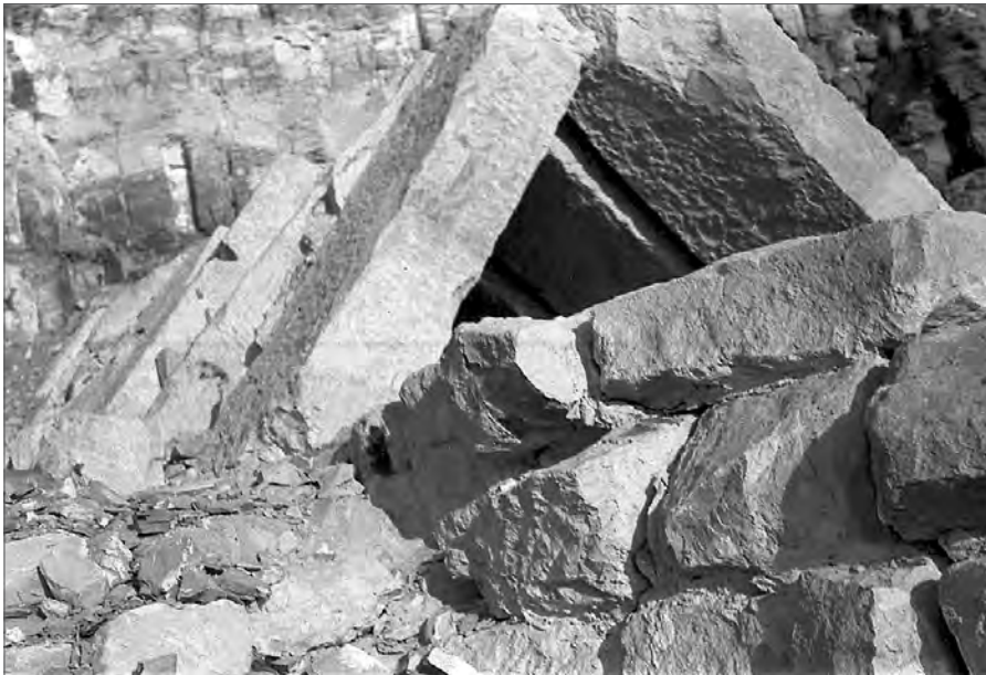
Fig. 1. Relieving structure above the Bark Hall of the Temple of Hatshepsut before undertaking restoration work (Photo © PCMA)
