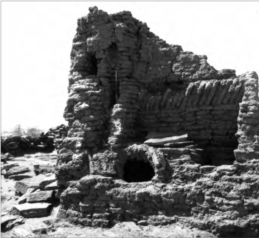
Fig. 10. Kumukka island. Core two-storey mud-brick building in settlement [16-S-5] (Photo ASSN F365/5)
