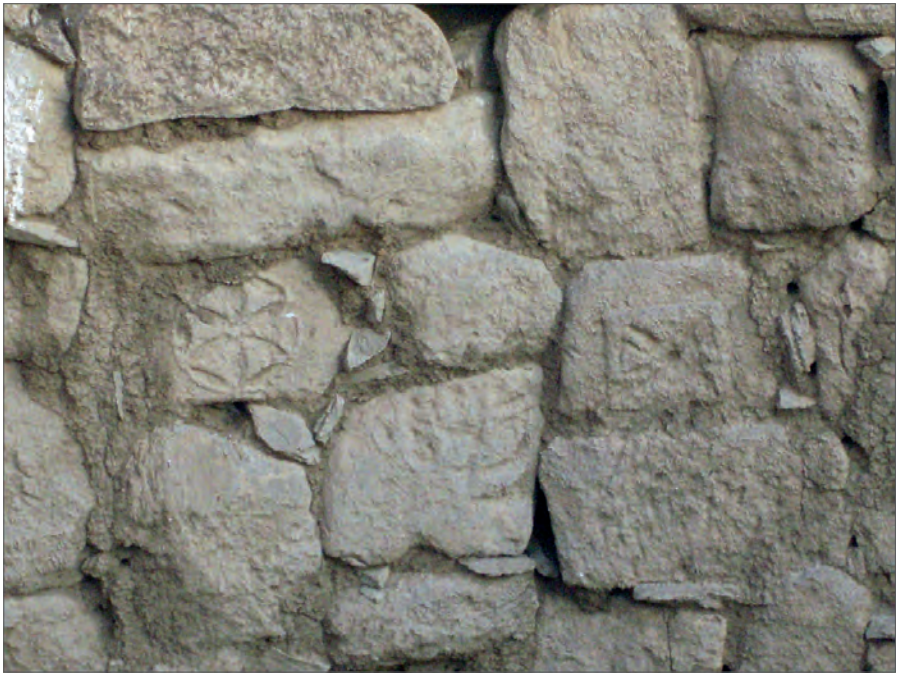
Fig. 8. Sandstone blocks with Christian decoration probably from a church and reused in the walls of a saqiyah well at site 8-B-500 (Photo H. Hafsaas-Tsakos)
