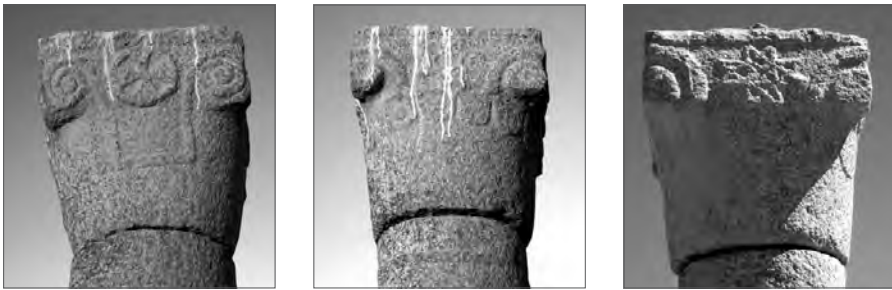
Fig. 7. Granite capitals from site 8-B-500: left, capital from the northeastern column, eastern face, style typical of that in the Church of Granite Columns at Old Dongola; center, capital from the southeastern column, eastern face with characteristic wreath of half-circles pending from the square upper part; right, capital from the southeastern column, western face, showing the unique equal-armed cross with v-shaped indentation of the arms (Photos H. Hafsaas-Tsakos)
