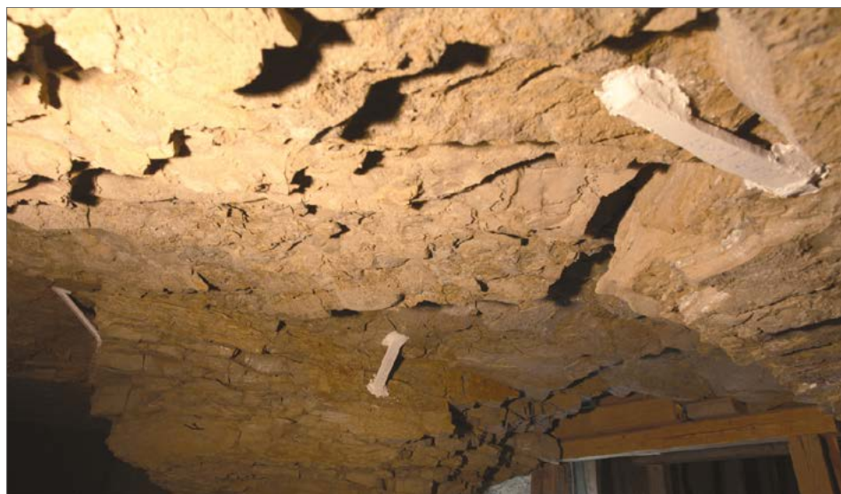
Fig. 8. Gypsum seals installed on the ceiling of the burial chamber of Chapel 32 (PCMA UW Saqqara Project/photo J. Dąbrowski)
