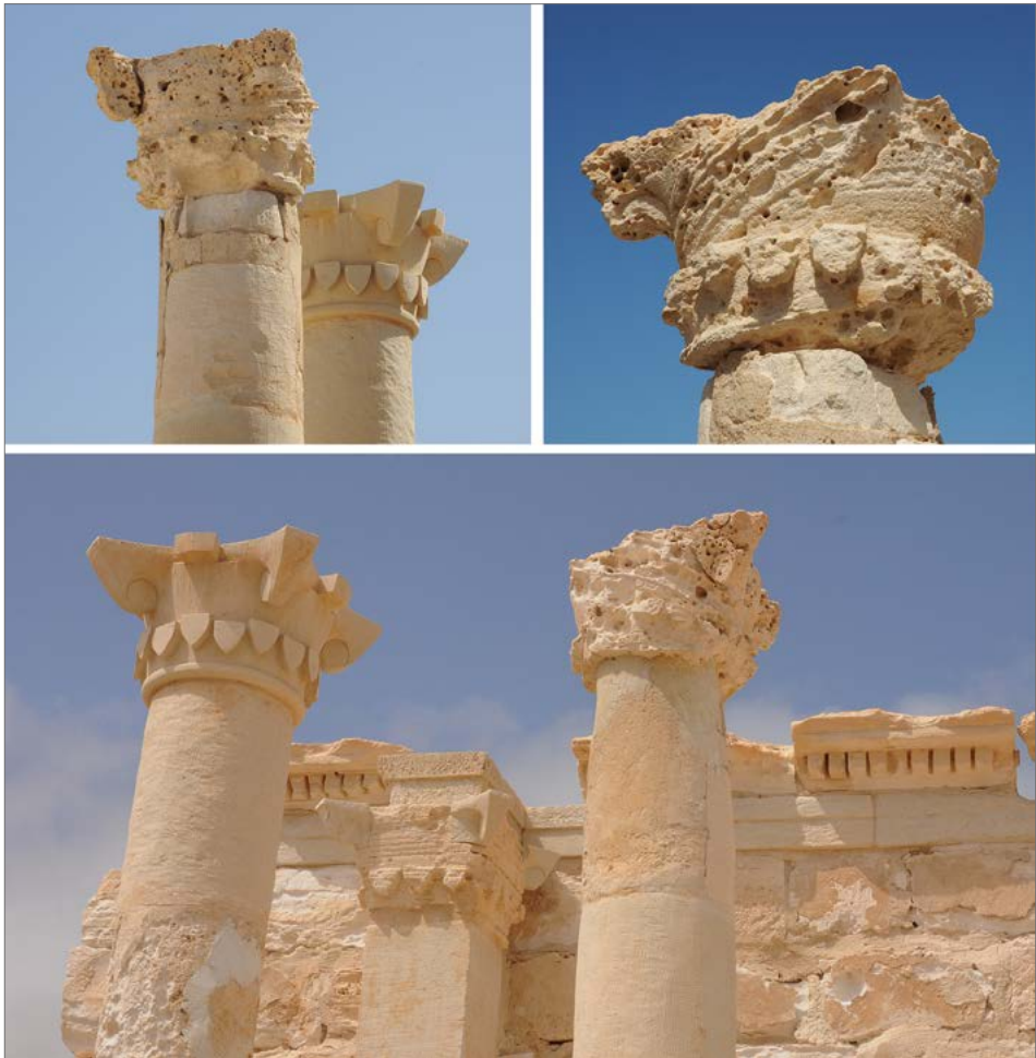
Fig. 2. Capitals of the commemorative monument in House H21: top row, before conservation; bottom, after conservation (Polish–Egyptian Conservation Mission Marina el-Alamein/photos P. Zambrzycki)
