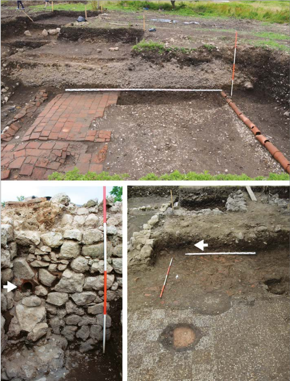
Fig. 5. Baths at Gonio: top, latrine floor (Phase 1) from east and water supply system consisting of ceramic pipes on the street north of the building (Phase 2); bottom left, northern edge of wall W2 viewed from the west, showing ceramic pipe for draining water from the frigidarium pool (Phase 1); bottom right, layer of broken roof tiles covering the mosaic floor from Phase 2, during exploration (Gonio/Apsaros Expedition/photos O. Kubrak, A. Trzop-Szczypiorska)
