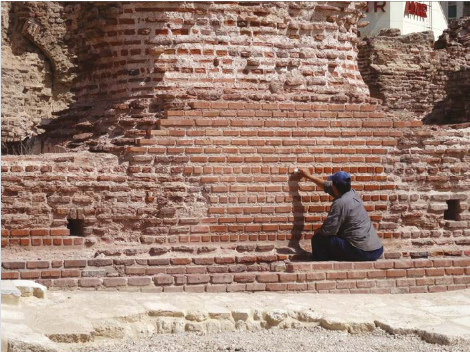
Fig. 15. Preservation work on the southern elevation of the late Roman Baths (PCMA Alexandria Kom el-Dikka Project/photo G. Majcherek)
