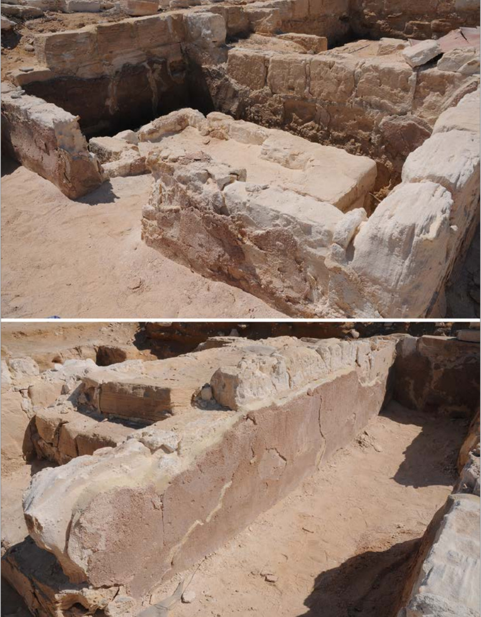
Fig. 3. Bands protecting ancient plaster edges in the Roman baths: top, before reconstruction; bottom, after reconstruction (Polish–Egyptian Conservation Mission Marina el-Alamein/ photos P. Zambrzycki)
