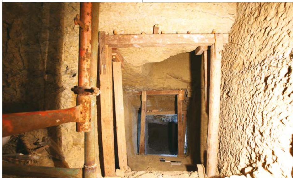
Fig. 3. Chapel 32: top left, state before exploration in 2015; center left, west wall with partly preserved blocking of the sloping corridor; bottom, steel and wooden supports in Chapel 32 and the sloping corridor leading to the burial chamber (PCMA UW Saqqara Project/photos J. Dąbrowski)
