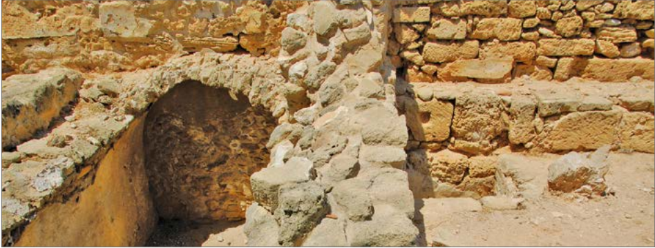
Fig. 3. Wall between rooms 13–15 on the left and 7 on the right, with plaster remains visible to the left and above the cistern (unit 15) and above a support wall in Room 7 (Photo E. Jastrzębowska, 2017)
