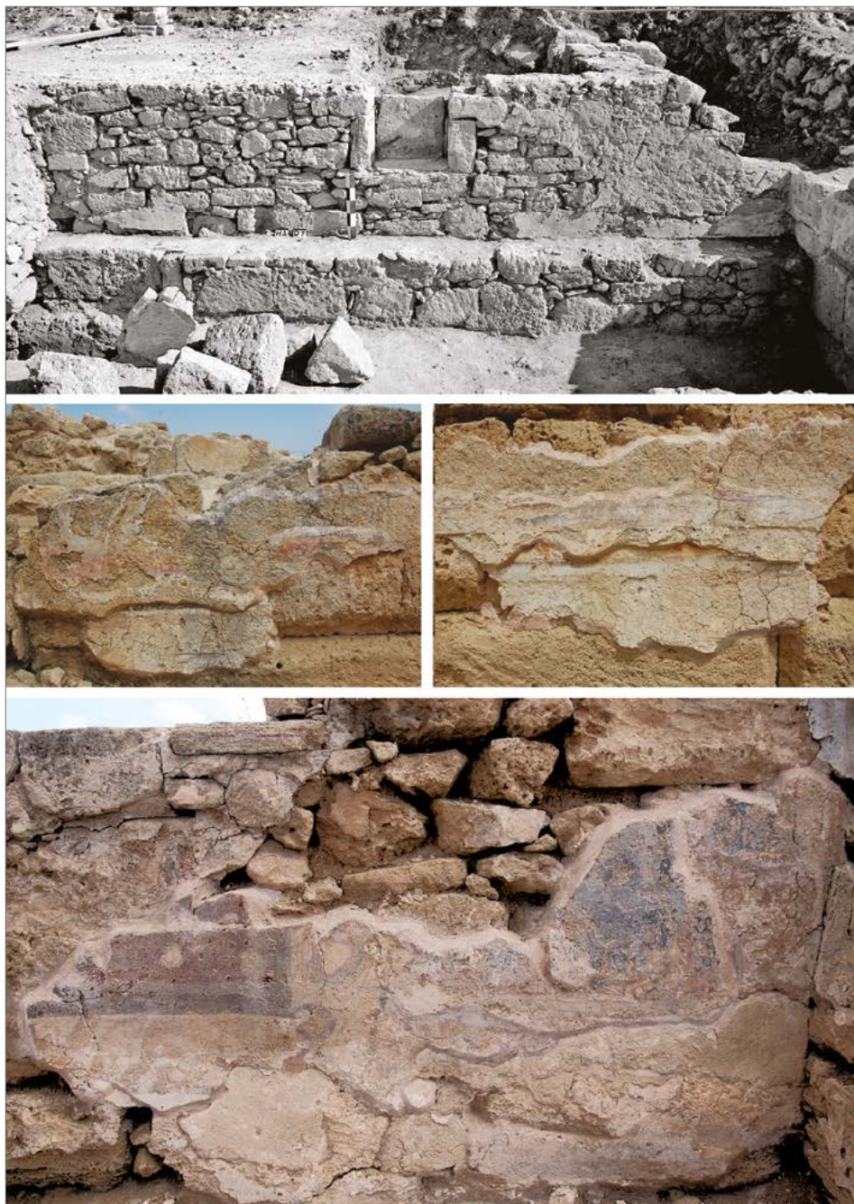
Fig. 11. Remains of painted plaster discovered still attached to the walls of Room 7: top, plain fragments on the north wall, touching directly on the surface of the support wall (1990); center, two layers of painted plaster on the northern end of the east wall; bottom, painted plaster in the western corner of the south wall (PCMA UW Nea Paphos Project/photos W.A. Daszewski, 1990; E. Jastrzębowska, 2017)
