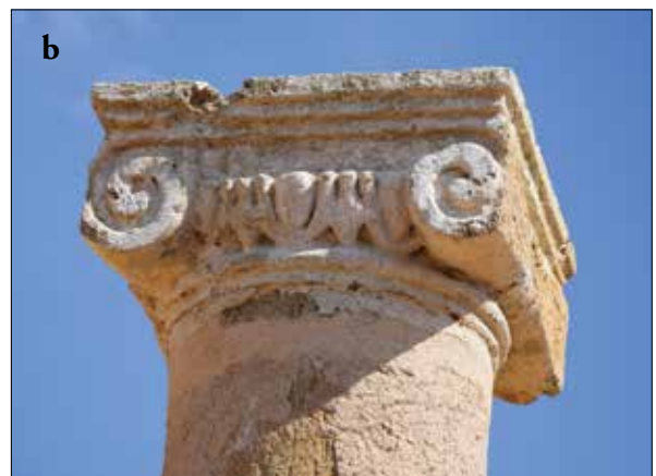
Fig. 24. Nea Paphos , 'Hellenistic' House, peristyle: a. Ionic colonnade; b. Ionic capital (photos by P. Pensabene).
