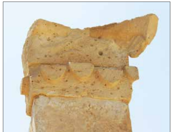
Fig. 7. Pseudo-Corinthian capital of the pillar framing the entrance from the courtyard to the prostas (photo by R. Czerner).
