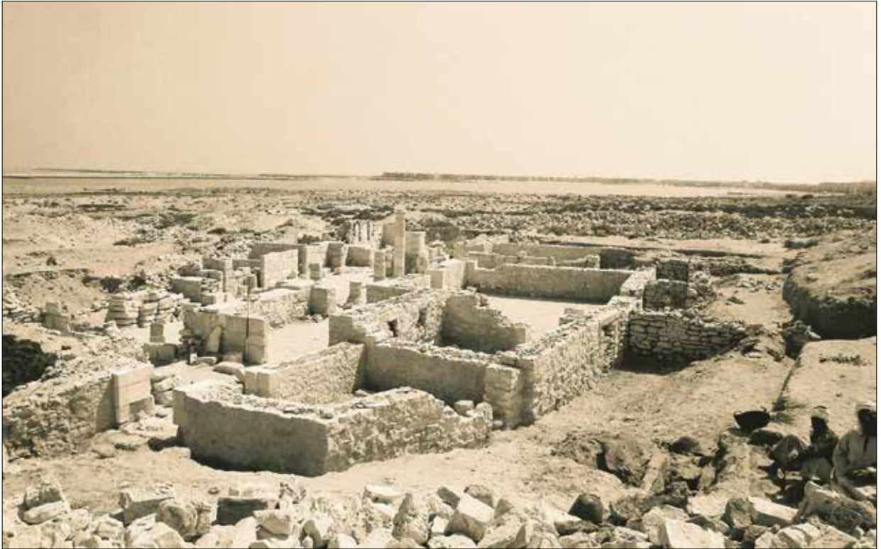
Fig. 3. Archival photo of House H9 during the conservation works in 1996, a view from the south-west (Archive of the Polish-Egyptian Conservation Mission).
