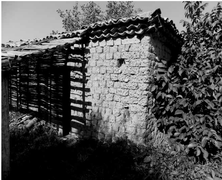
Fig. 1. A modern mudbrick structure in Greece that possesses many of the features of the prevailing vernacular methods in the region (photo by K. Jazwa).
